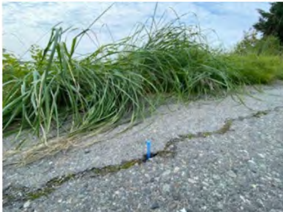
Figure 3-55 Pavement Cracking on Max Italio Dr. (2022)
