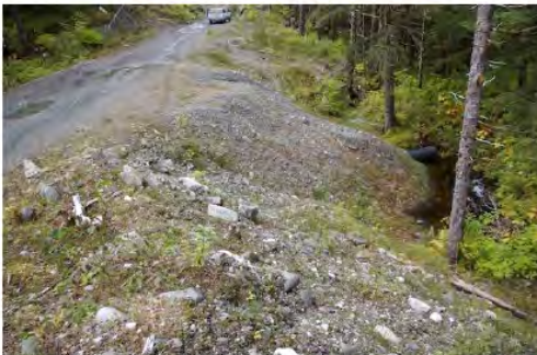
Photo 3: Erosion on inland subdivision road, September 2007.
