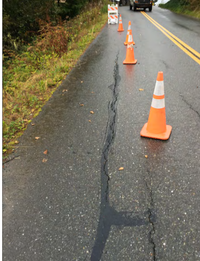
Figure 3-50 Creeping Slope Failure of Max Italio Dr. (August 29, 2016)
