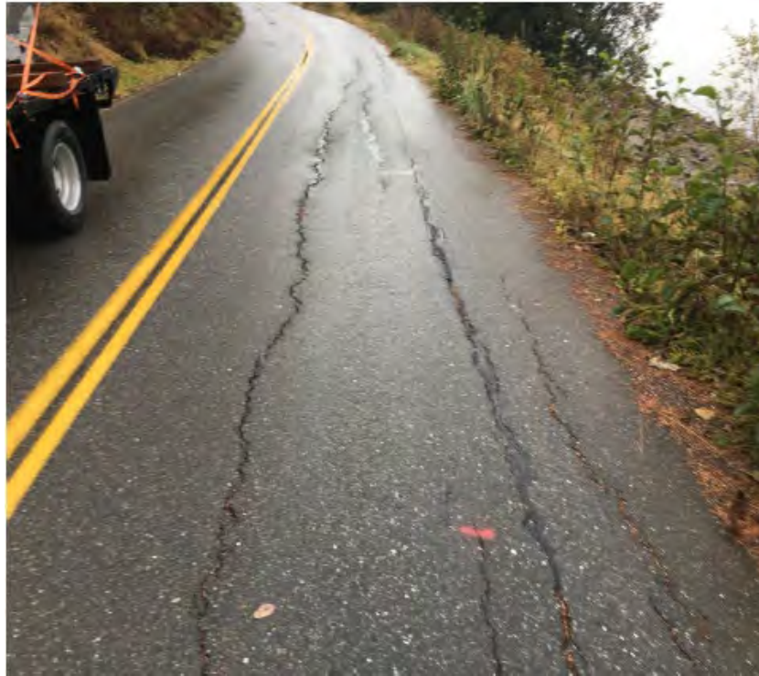
Figure 3-55 Pavement Cracking on Max Italio Dr. (2022)
