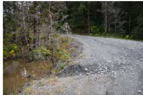
Photo 4: Erosion on inland subdivision road, September 2007.
